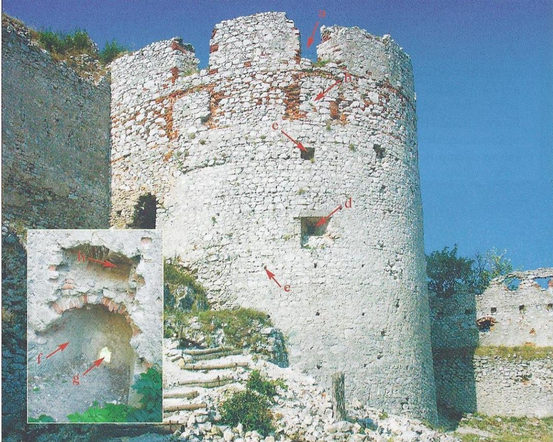
Picture 6 - cannon turret of the upper castle, a – shooting position, b – walled in shooting position, c – ventilation channel, d – cannon shooting position, e – opening left behind after wooden scaffolding, f – chamber shooting position for cannon, g – shooting position opening, h – ventilation channel
