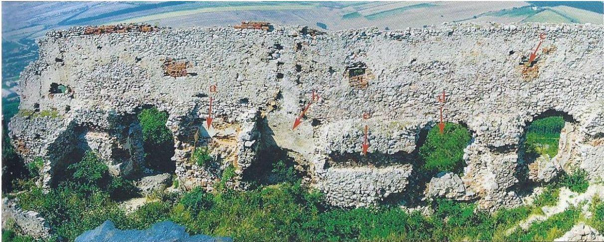
Picture 8 – housing building of the upper castle, a – walled in alcove, b – furnace with chimney, c – remains of arches of the 2 nd story, d – windows of the 2 nd story, e – windows of the 3 rd story
