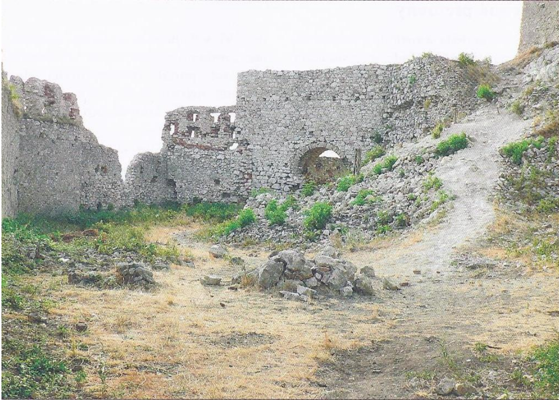
Southern castle outwork court, with entry gate in the background
