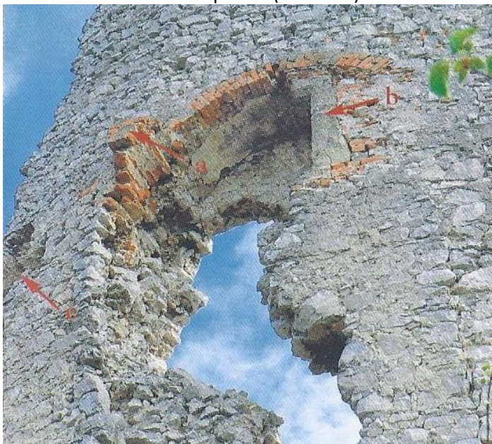
Picture 3 -Northern wall of the castle palace, a – remains of the prevét, b – remains of the palace gothic window, c – crenel of the walled in battlement of the original wall
