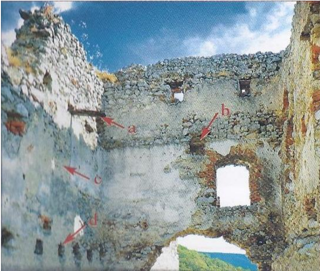
Picture 1 - room above the gateway of the entry gate tower, a – remains of the beam ceiling of the 2 nd story, b – beam supporting the walling, c – furnace, d – seats remaining after beams of the original 1 st story ceiling.
